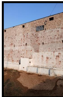
3c- i. Cow feed storage with Iron shed and Gate constructed at Shiv Krishan Gaushala on Sandawa Road, Bidasar , in the year 2025
