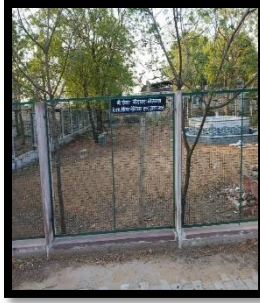
MUKTI DHAM 4b- Iron structure of Boundry wall of the garden
