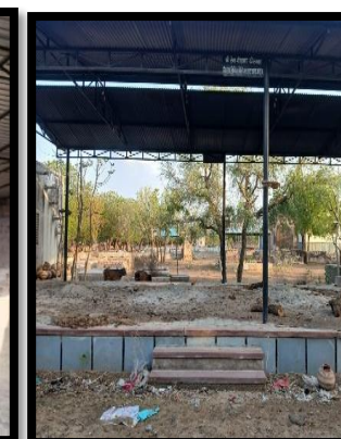
MUKTI DHAM 4a- i. Reconstruction of the structure and Shed
