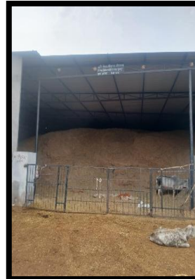
3a- ii. Cow feed storage with Iron shed and Gate constructed at Shree Ganesh Gaushala on Shree Dungargarh Road, Bidasar , in the year 2021
