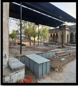
MUKTI DHAM 4a- ii. Reconstruction of the structure and Shed
