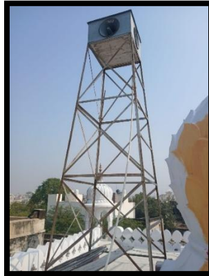
6. Mike and Sound system Recently,in October, 2025,installed at a very much prominent Shree Ramdev Ji mandir,Dhanawato Ka Mohalla,on the way to Balbari School from SBI.
