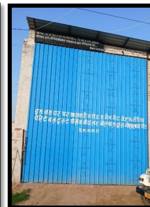
3c- ii. Cow feed storage with Iron shed and Gate constructed at Shiv Krishan Gaushala on Sandawa Road, Bidasar , in the year 2025
