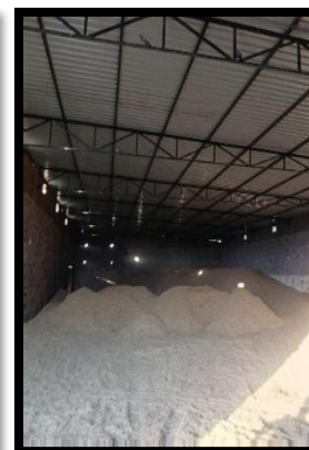
3c- iii. Cow feed storage with Iron shed and Gate constructed at Shiv Krishan Gaushala on Sandawa Road, Bidasar , in the year 2025
