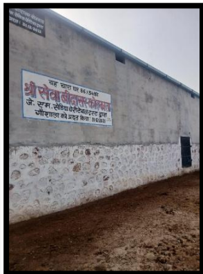
3a- i. Cow feed storage with Iron shed and Gate constructed at Shree Ganesh Gaushala on Shree Dungargarh Road, Bidasar , in the year 2021
